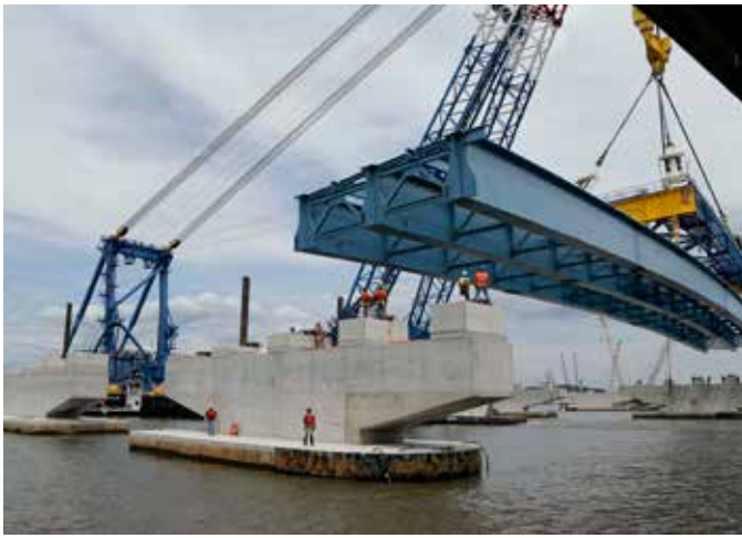
The Tappan Zee Bridge under construction in New York.
