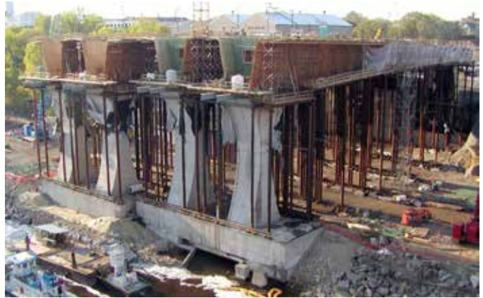
St. Anthony Falls Bridge under construction. (Wikipedia)
