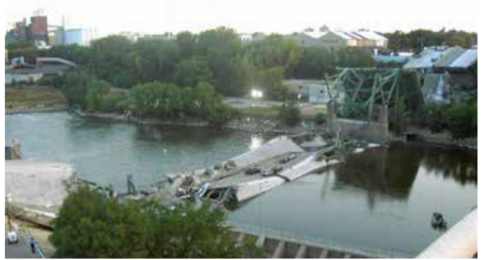
The St. Anthony Falls Bridge in Minneapolis, MN collapsed in 2007. (Wikipedia)
